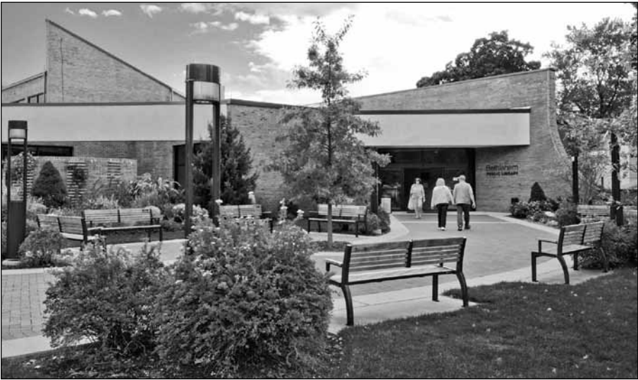
The entrance gardens today ( Bethlehem Public Library archives )
