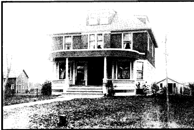
Home of William A. and Nettie Vanderzee Glenn in Elsmere. Built by John Vanderzee, ca. 1905.
