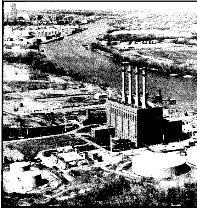
The Niagara Mohawk station in Glenmont.
